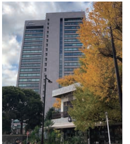
The Itochu Corporation building will be rebuilt to nearly twice its current height.
